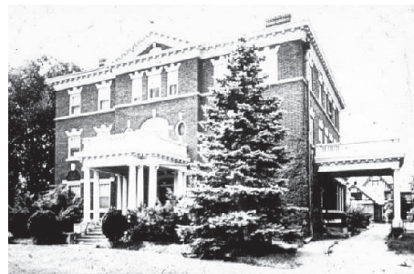
This magnificent home, the Richardson House once stood at the corner of Collingwood and Floyd.
